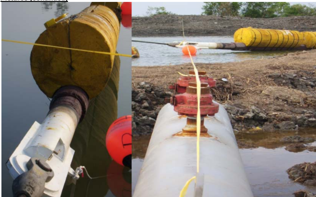
Pipeline pulling head at target location
