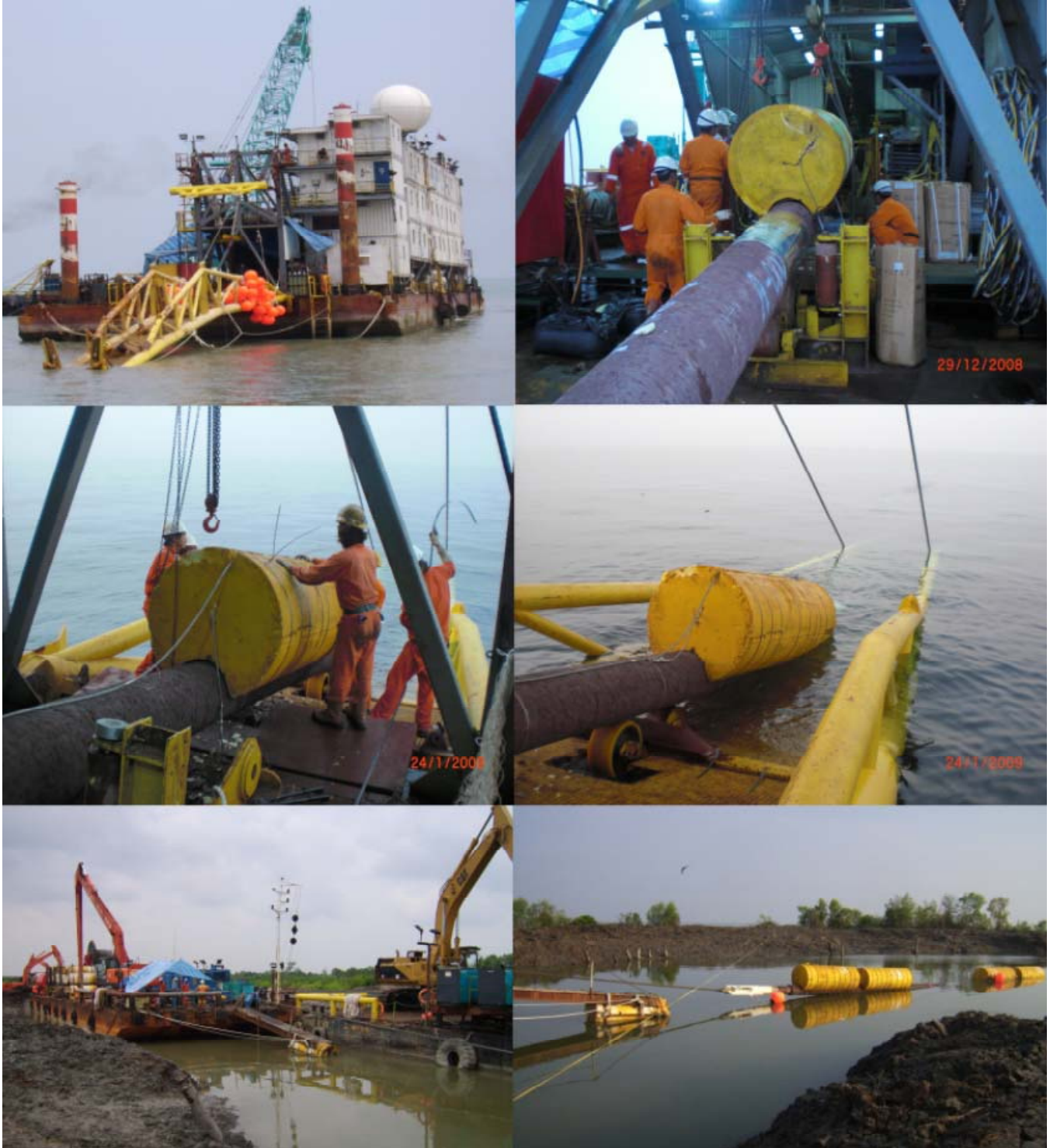
Pipelay barge and buoyancy attachment, pull barge with head arrival
