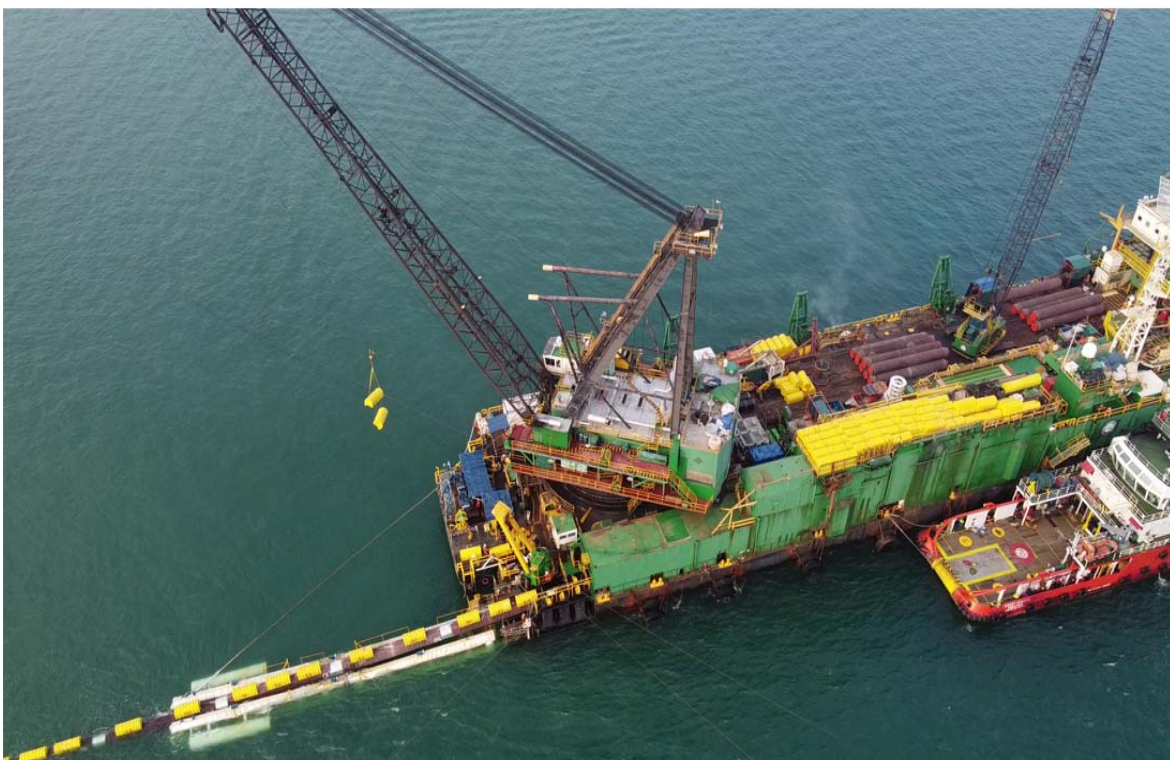
Beach pull / pipelay using DLB01
