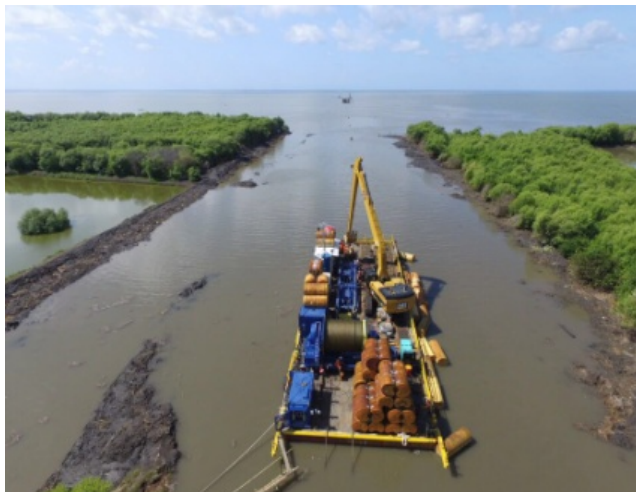
PRE TRENCH AND PULL BARGE
