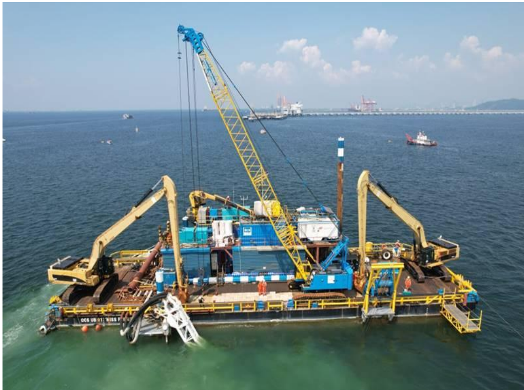
Figure 8.5.6 Pre-Trenching with Trailing Arm in Sriracha Project
