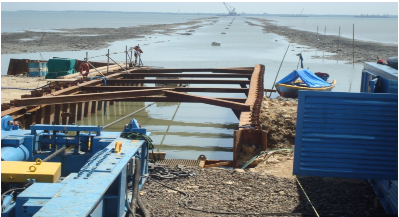
BEACHPULL OPERATION AND COFFERDAM
