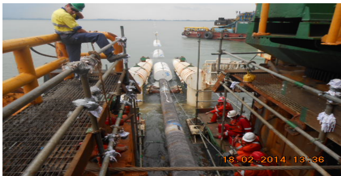
BEACH PULL / PIPELAY FROM PIPELAY BARGE DLB01)
