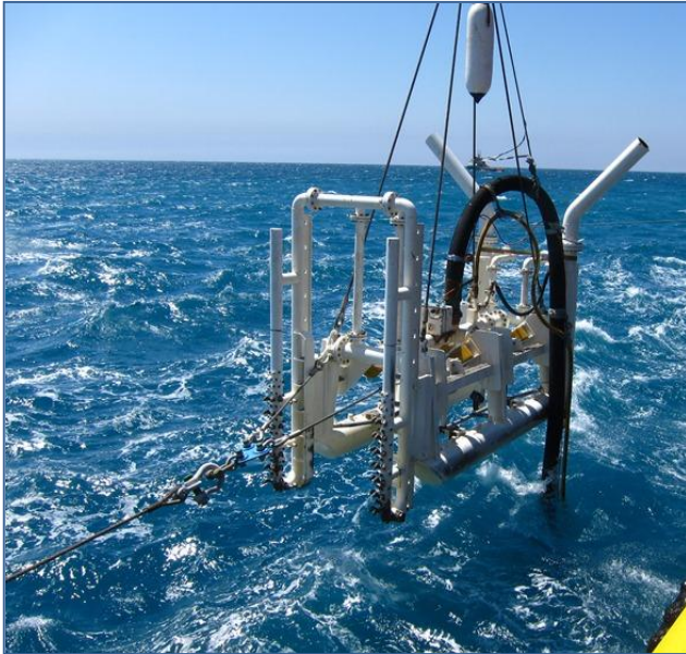
Figure 9.11.1 Setting SLED onto pipeline
