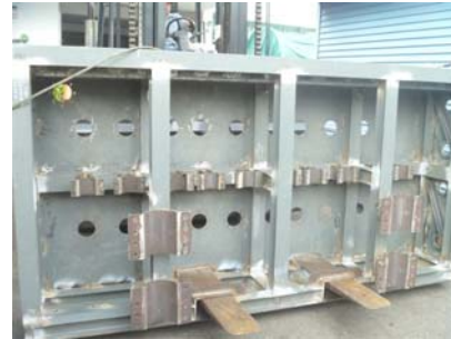
Fabrication of SSU skid frame
