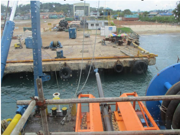
Tensioner Paying Out Test Pipe
