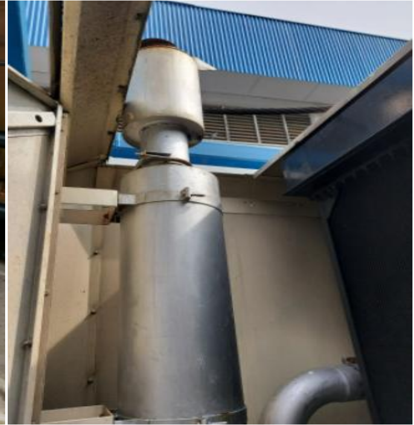
Exhaust System complete with Spark Arrestor
