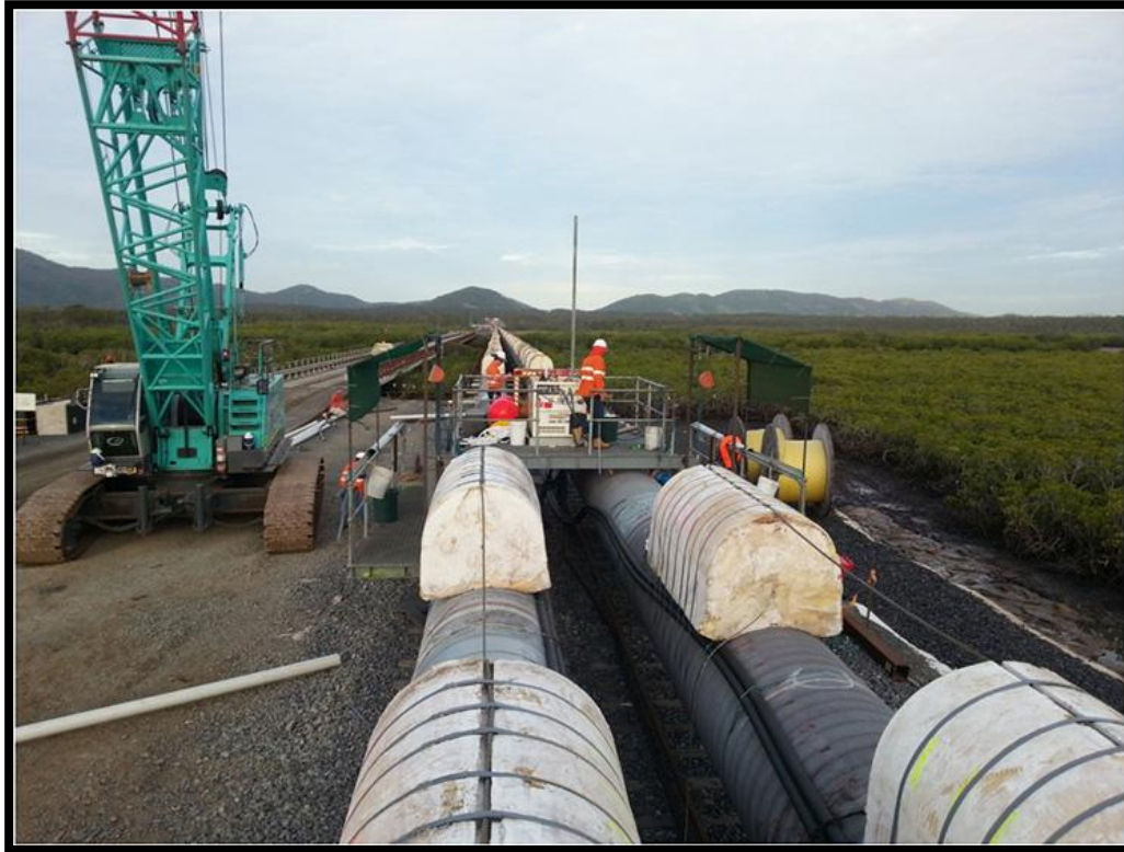
Foam Buoyancy Installation
