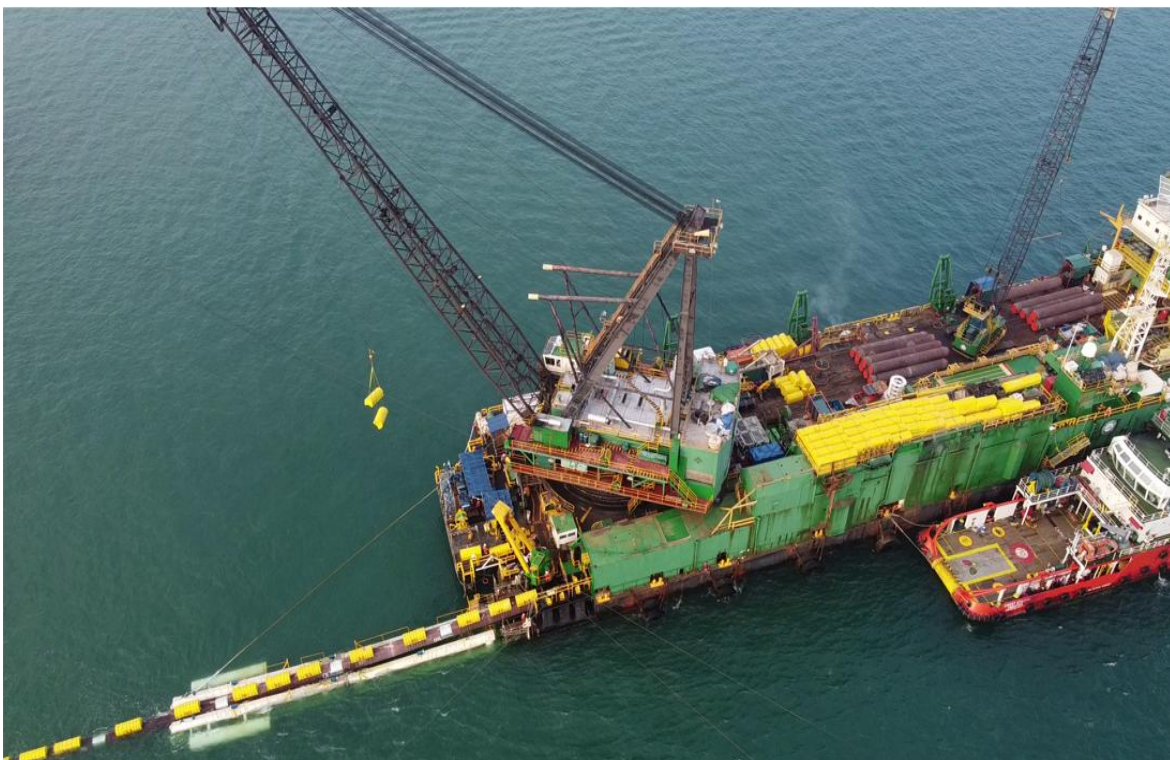
Beach pull / pipelay using DLB01
