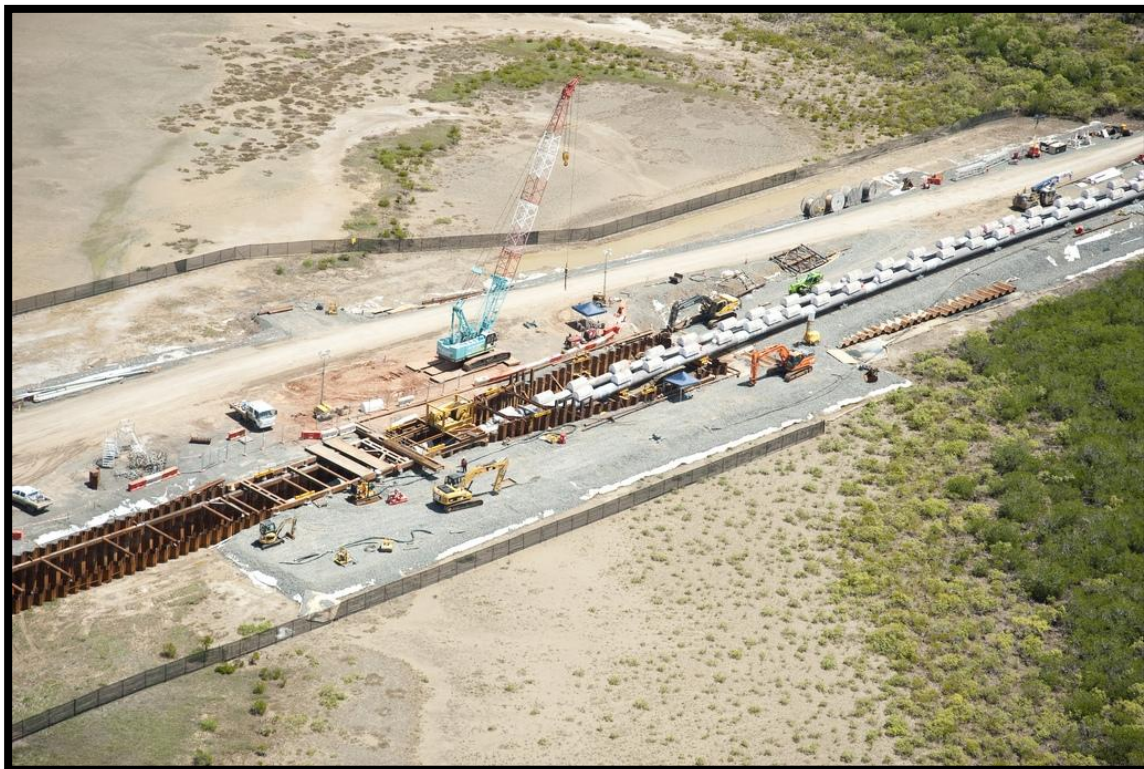
Pipe-pull into cofferdam
