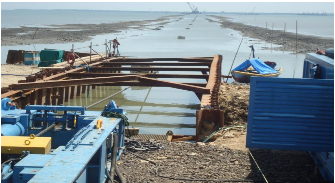
BEACHPULL OPERATION AND COFFERDAM
