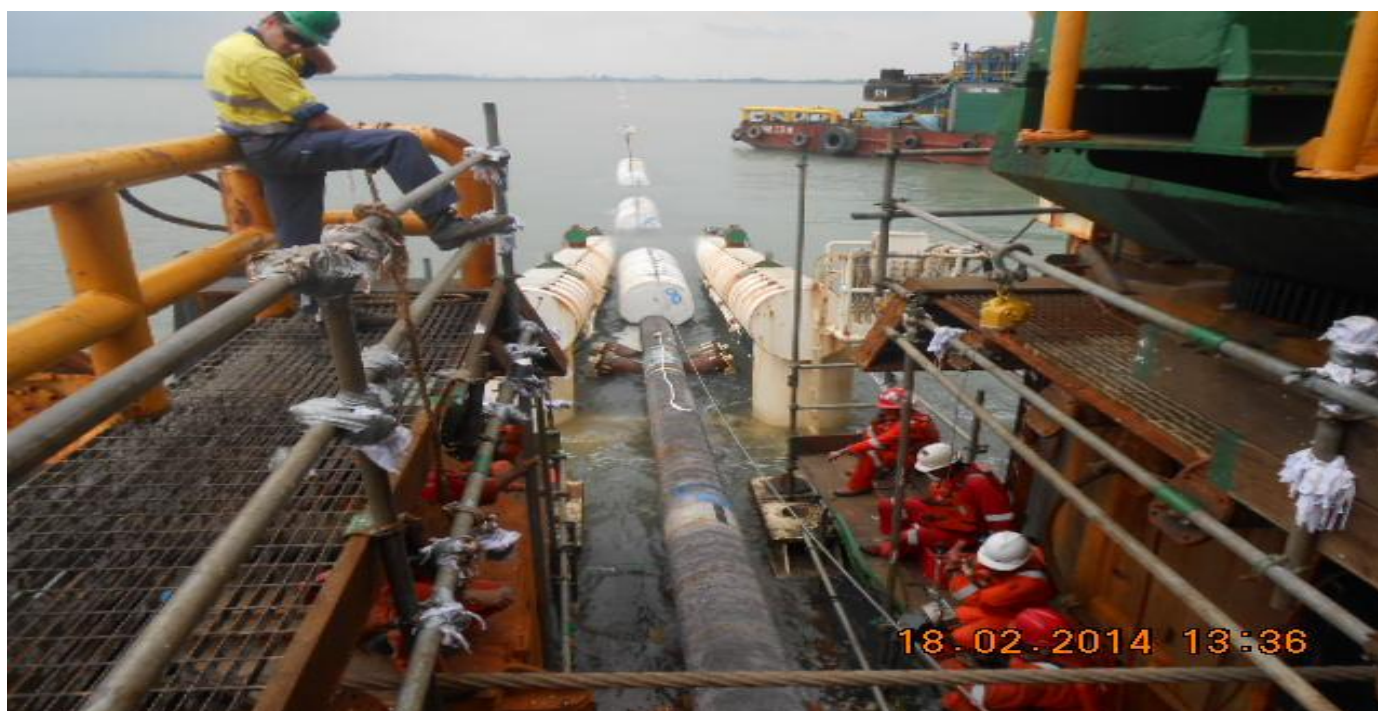
BEACH PULL / PIPELAY FROM PIPELAY BARGE DLB01)
