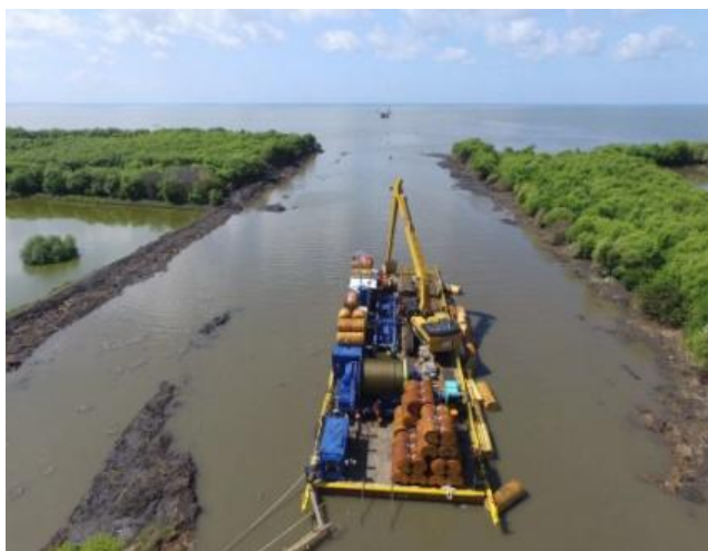
PRE TRENCH AND PULL BARGE
