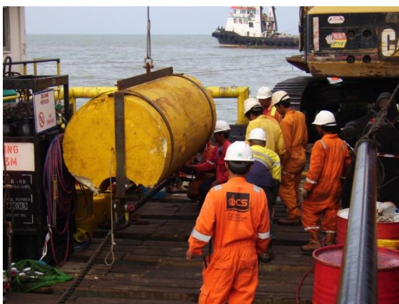
Pull Cable buoyancy
