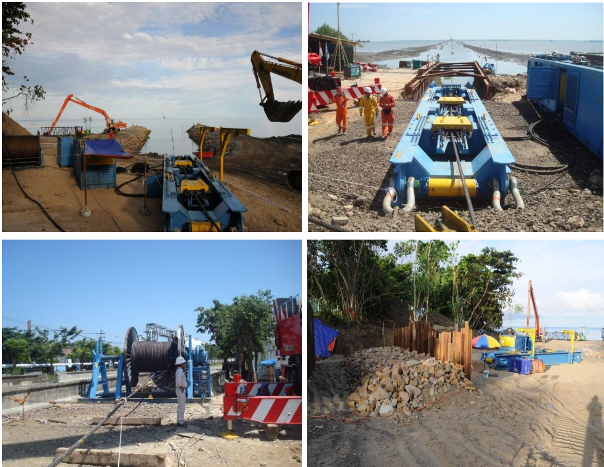
Figure 4.4.1 Typical Lucker Winch/Spooler set up on the beach head
