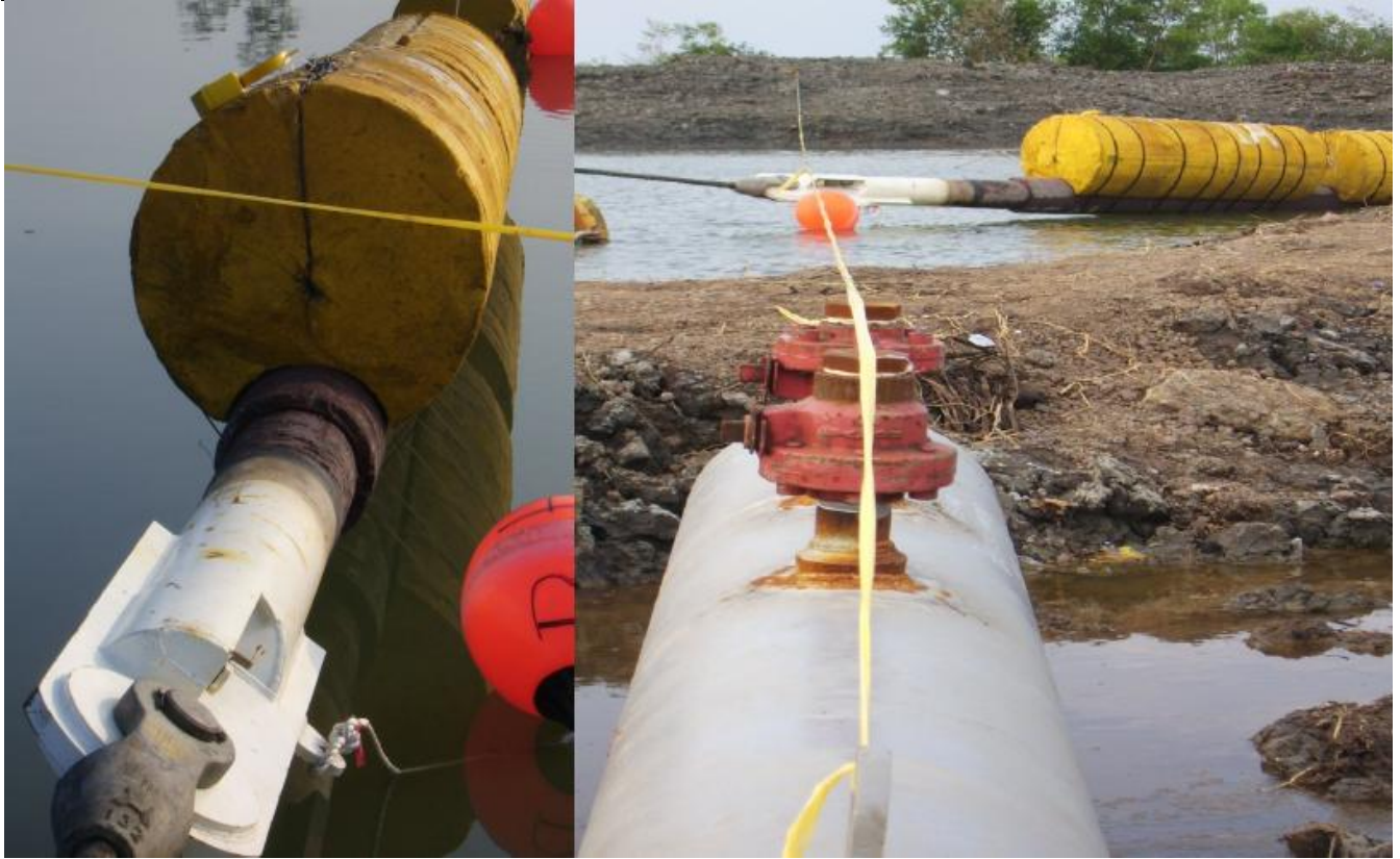
Pipeline pulling head at target location
