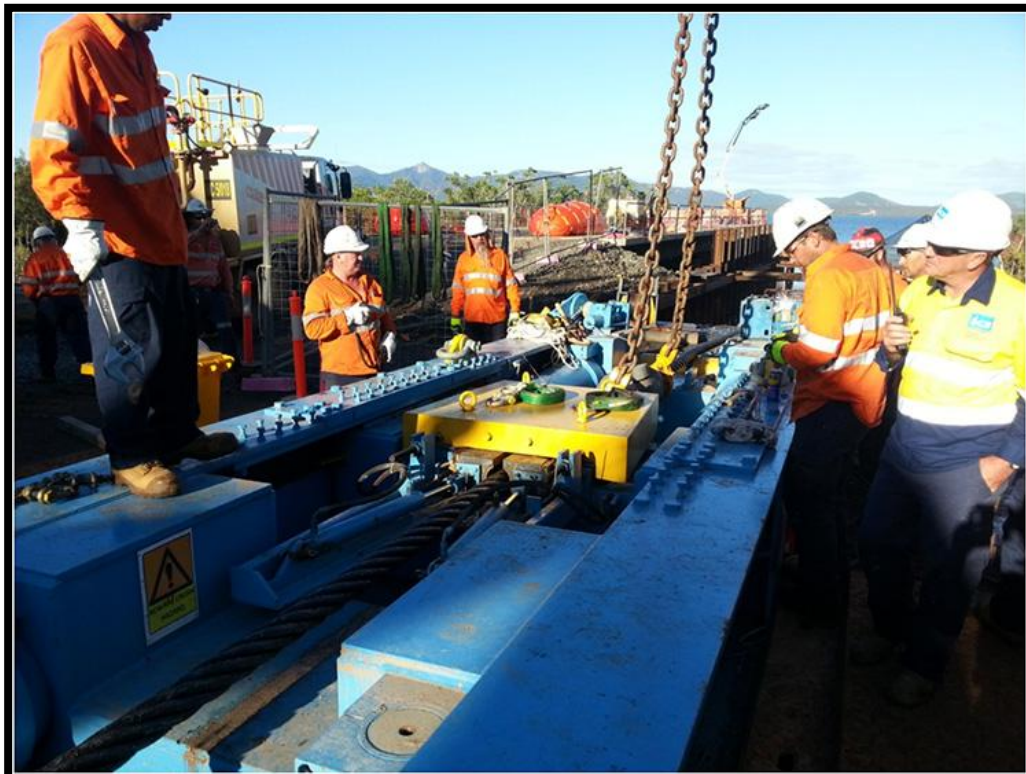
In-hauling of pipe string with Linear Winch Puller
