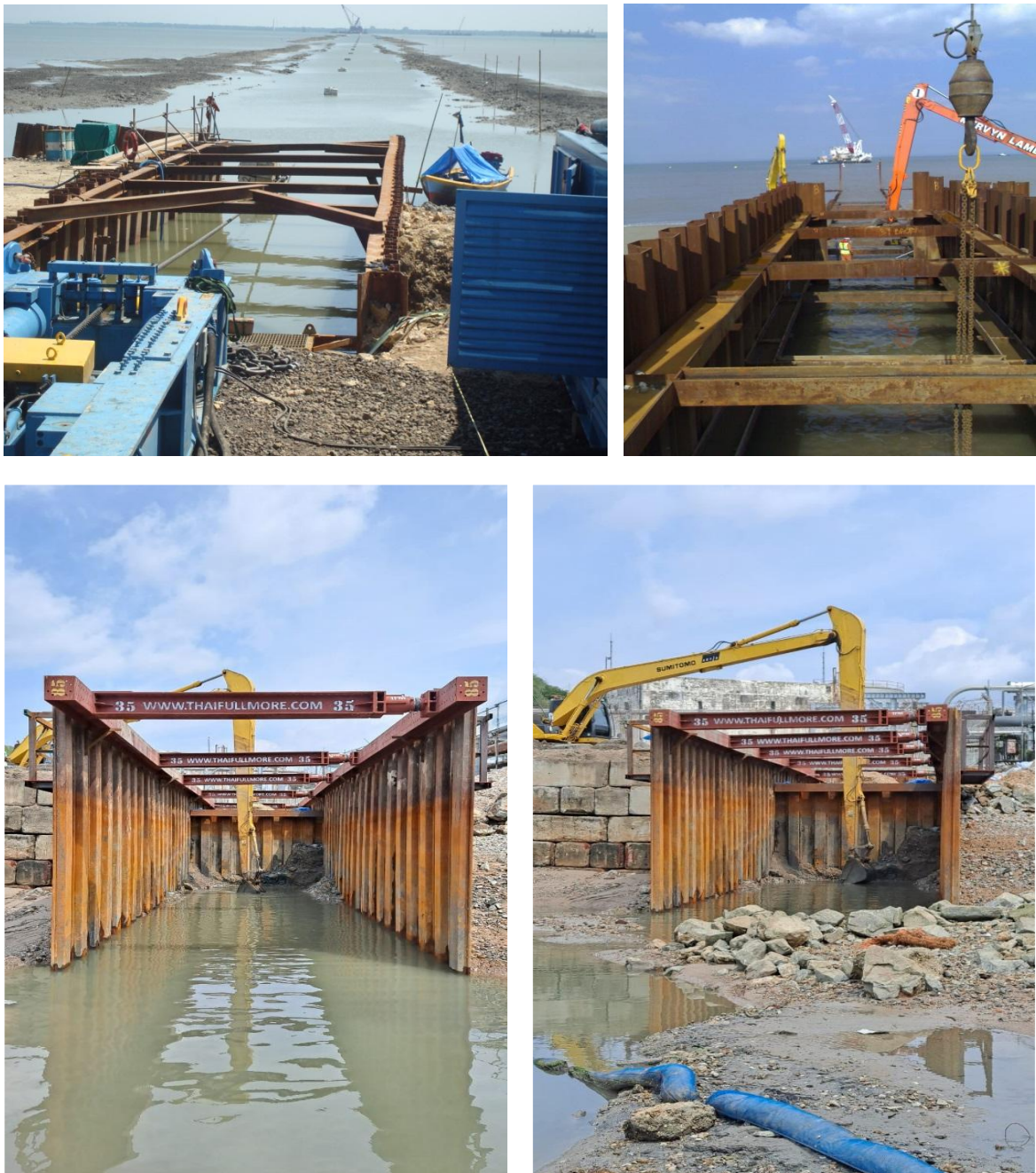
Figure 4.3.1 Typical cofferdams (previous projects)
