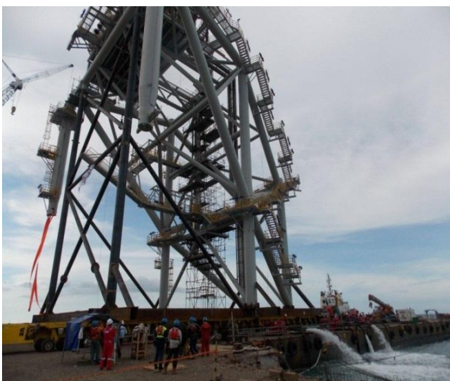
Marine Support Structure Loadout
