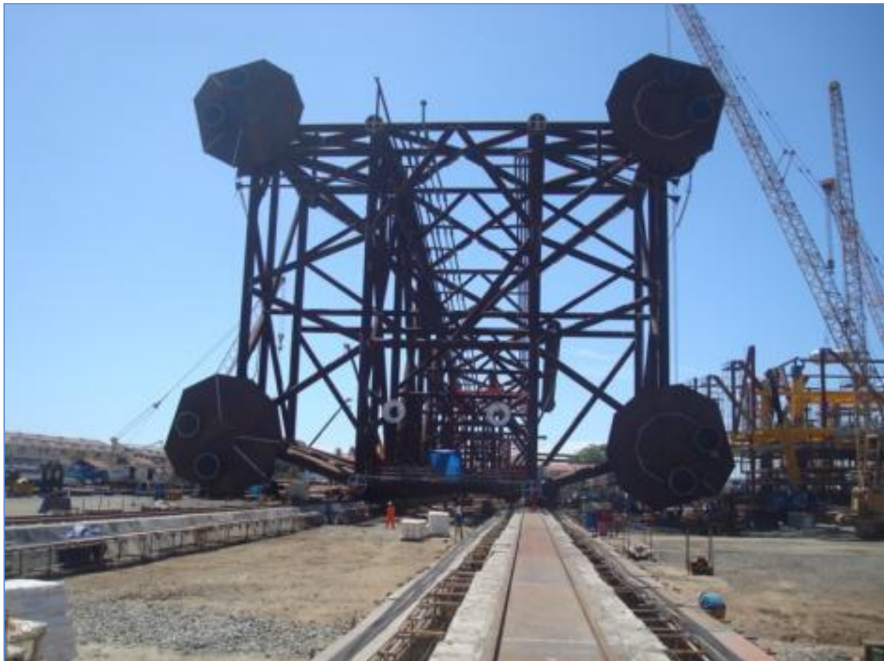
DH2 jacket being loaded out
