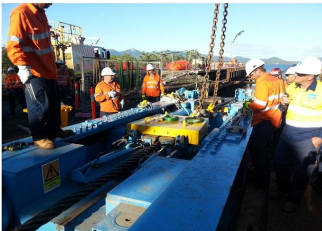
In hauling pipestring with Linear Winch Puller
