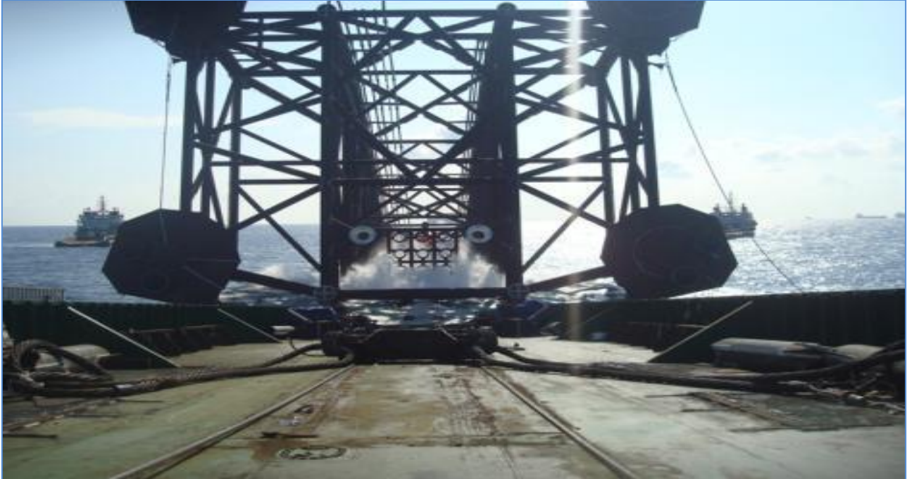
DH2 jacket launched coming off launch barge VSP05
