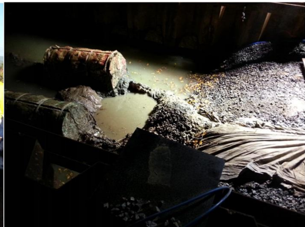
Pullhead making landfall
