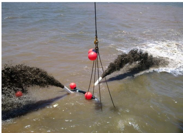
Shallow Water Jetting in Progress
