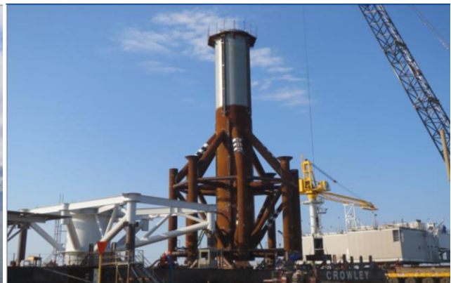
Monopod Loadout at SSCI Yard
