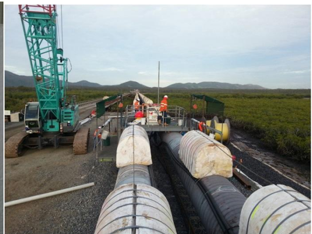
Foam Buoyancy Installation onto pipestring
