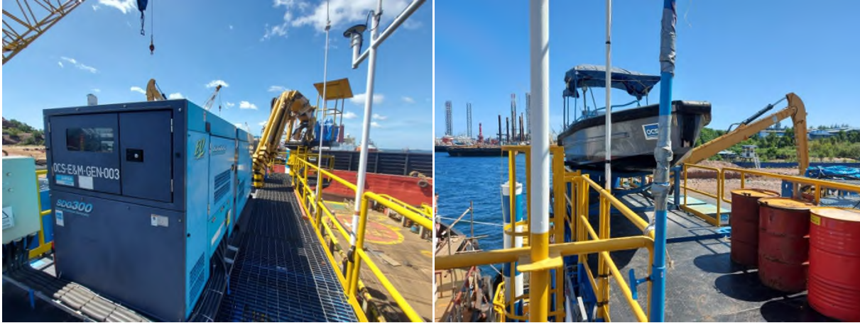
Figure 3-8 Generator & Knuckle Boom and Dive Support Boat
