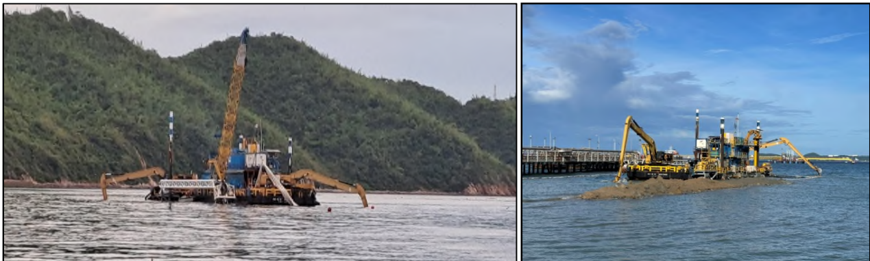
Figure 4-2 UB-01 Pre-trenching with Excavators in Sriracha Project (Thailand)
