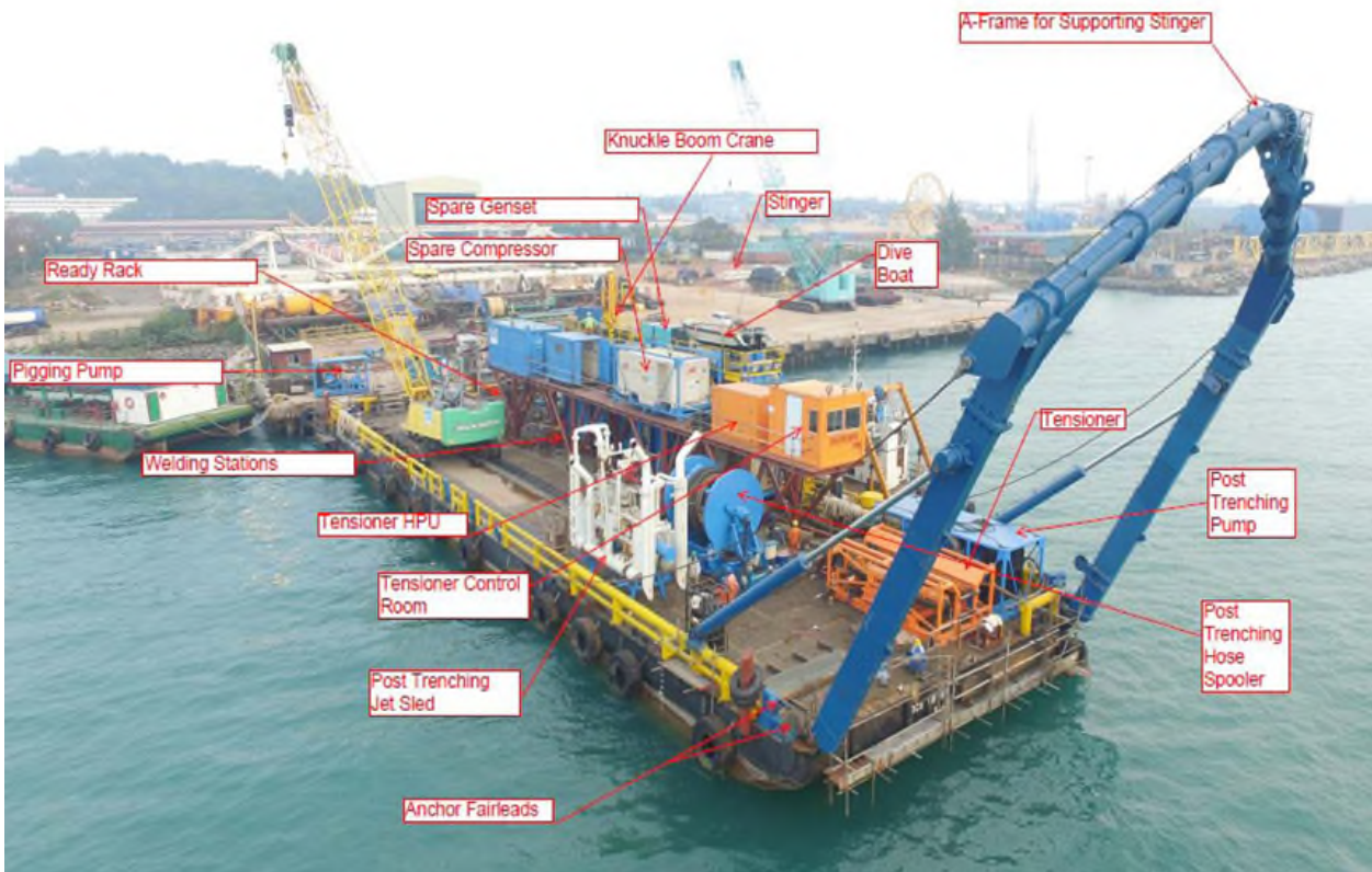
Figure 3-2 General View of Miss Pennie – Configured for Pipelay (Stinger not installed)
